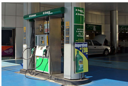
Ethanol pump station in São Paulo, Brazil
